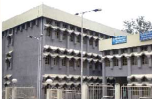
Physics Department Building
